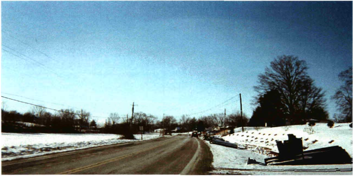
LOOKING SOUTH ON SR 134 / 800 FEET FROM INTERSECTION
