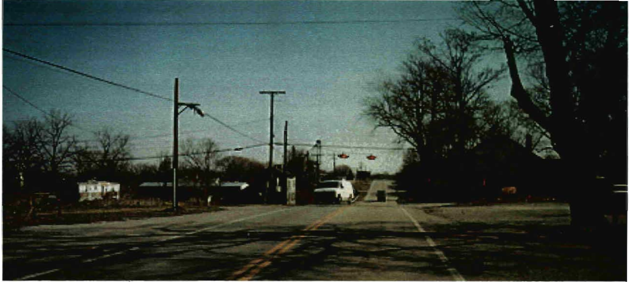
LOOKING EAST ON USR 50 200 FEET FROM INTERSECTION
