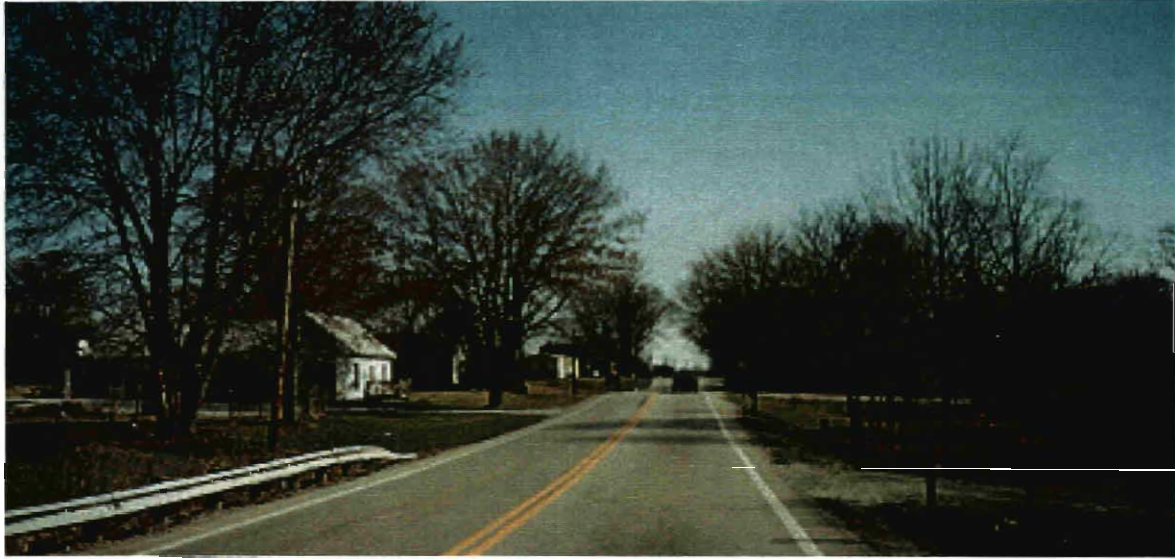
LOOKING EAST ON USR 50 1,000 FEET FROM INTERSECTION
