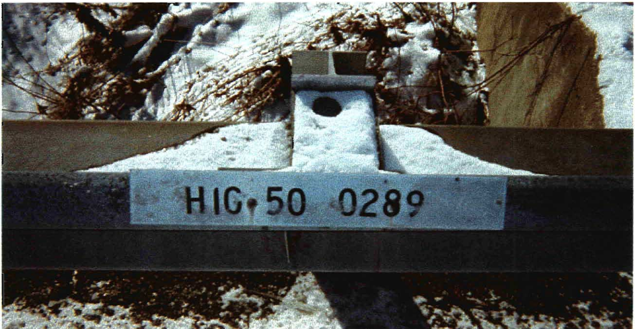
CULVERT ON US 50, EAST OF PROJECT
