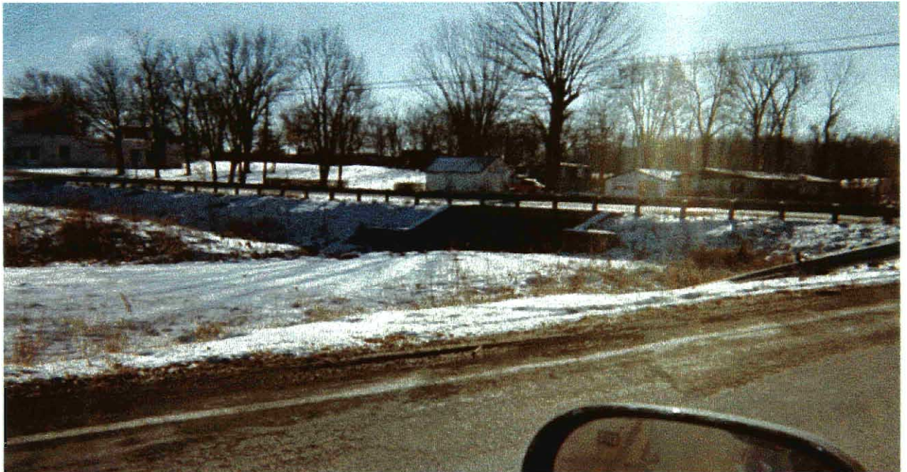
CULVERT ON US 50, EAST OF PROJECT
