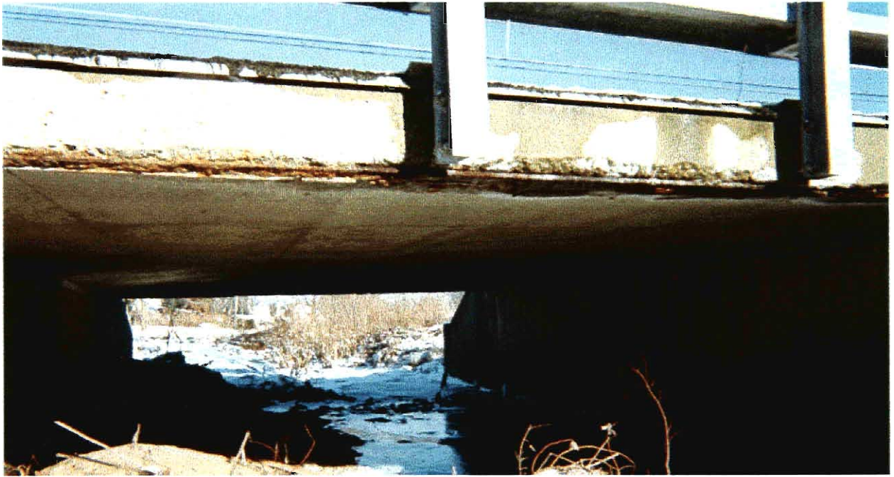
CULVERT ON US 50, EAST OF PROJECT
