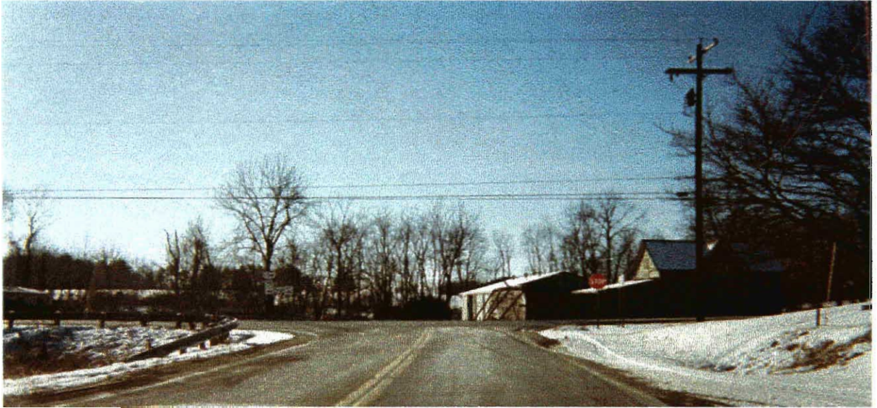
LOOKING SOUTH ON SR 134 / 100 FEET FROM INTERSECTION
