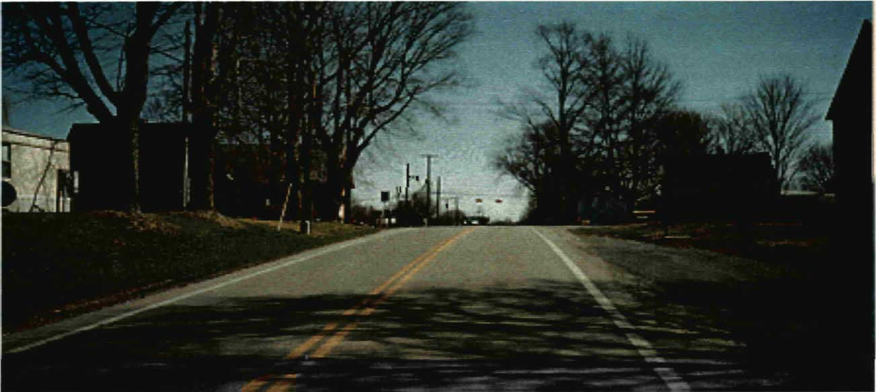
LOOKING EAST ON USR 50 400 FEET FROM INTERSECTION
