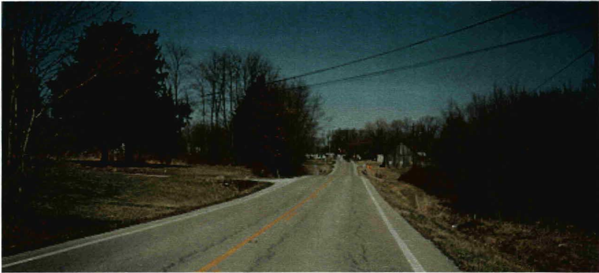
LOOKING NORTH ON SR 134 1,000 FEET FROM INTERSECTION
